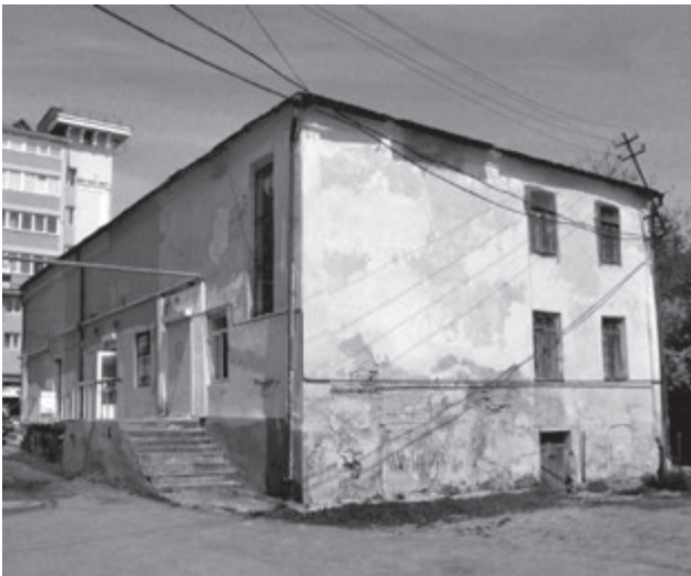
Fig. 24. The Tailors' Prayer House, view from southwest. Photo by S. Kravtsov, 2011. CJA
